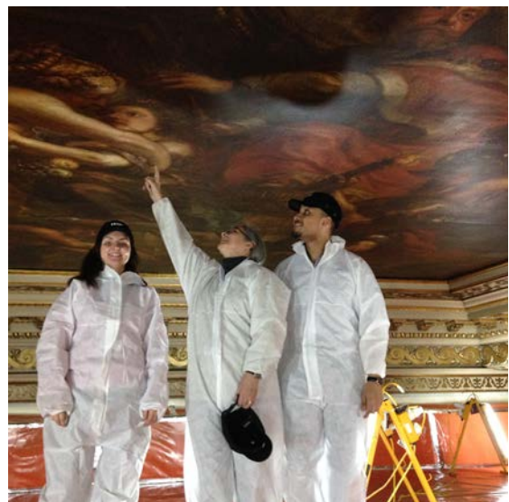
Figure 14: The BH project team take advantage of the scaffold access, before the asbestos work begins above, to get a close up view of the Rubens paintings
