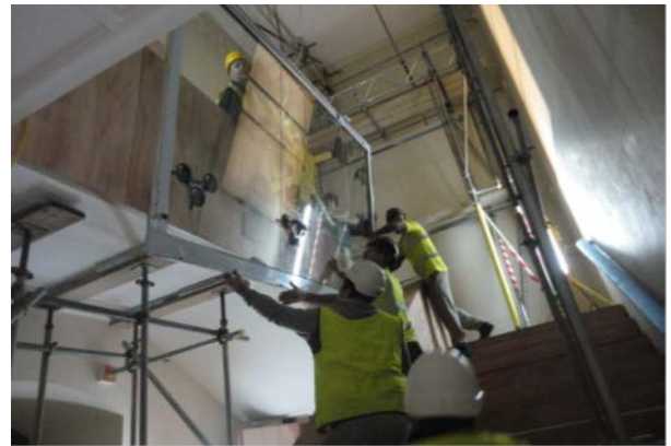
Fig. 10 Lifting the windows on to the first floor
