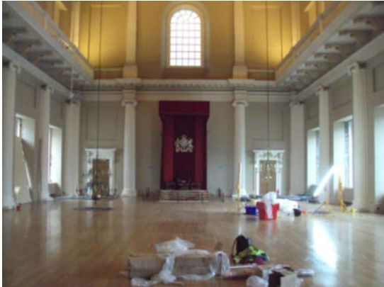
Figure 3: Clearing the hall and removing the window protections
