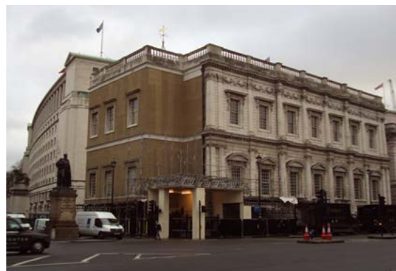
Figure 1: Scaffold struck to below Gantry Level
