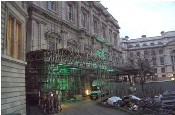
Fig. 2: Scaffold strike at rear of building
