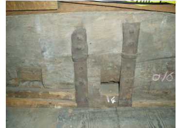
Lowered floor level, hung off principal beams.
