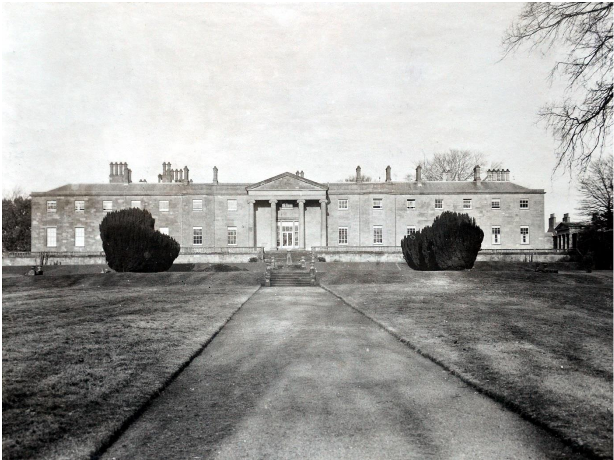
South Façade at Hillsborough Castle, circa 1926
